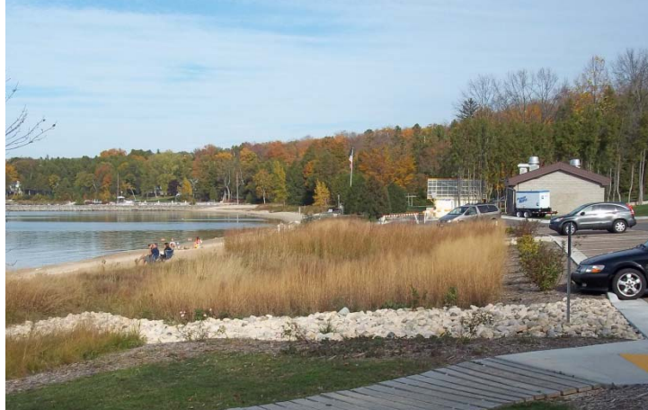
Infiltration swale vegetated with native grasses
