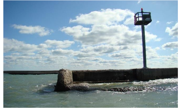
The end of the North Pier shows the spalling concrete and exposed rebar near the coast guard light.
